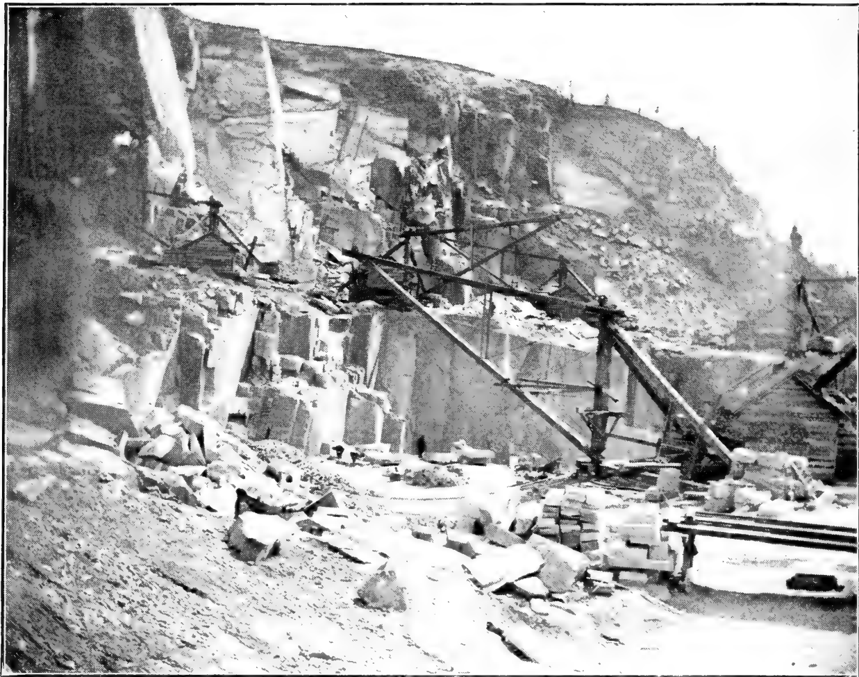
FIG. 1.—McClenahan & Brother's quarry, showing jointing in the granite-gneiss.
