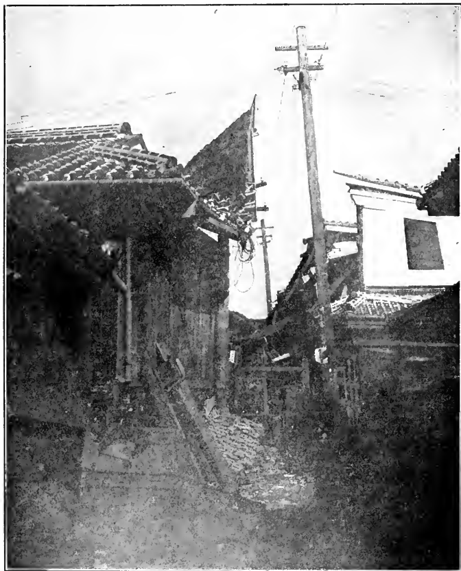
FIG. 17.—Houses in Kagoshima damaged by the earthquake. (Photo taken on Jan. 16.)
