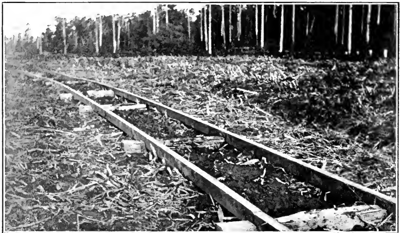
TRAM TRACK, MESSRS. HALFORD BROS.' FARM, KONGWAK.
