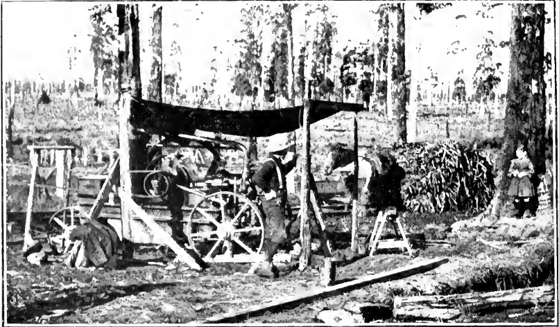
OIL ENGINE AND LOADED TRUCK.
