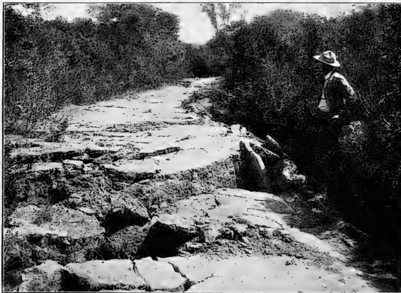
FIG. 3.—Road crossing the fault-line two miles southeast of Portola. There is a vertical uplift on the northeast side of the fracture at this place.
