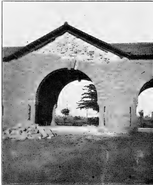
FIG. 9.—Photograph of arches at Stanford University, showing keystones lowered during the earthquake. These arches were nearly at right angles to the fault-line.
