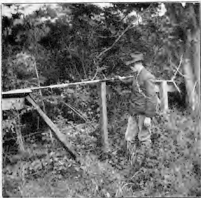
FIG. 4.—Showing a fence that crossed the fault at an oblique angle. The post shown in the photograph was split and pulled apart and the wires broken.
