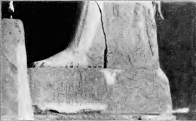
FIG. 3.—Statue of Rameses II. Entrance to the Great Hypostyle Hall, Karnak, showing in a characteristic manner the exfoliation of the pedestal, feet, and lower legs.
