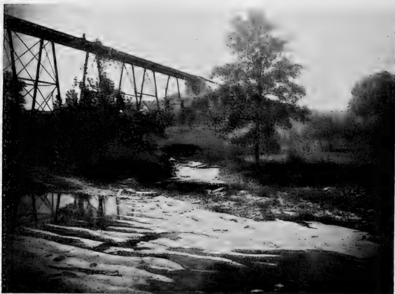
FIG. 1.—View of ripple-marks in bed of Elk Run, just below the Norfolk & Western Railway trestle, 1\frac{1}{4} miles east of Winchester, Ohio. Photograph by C. S. Prosser.
