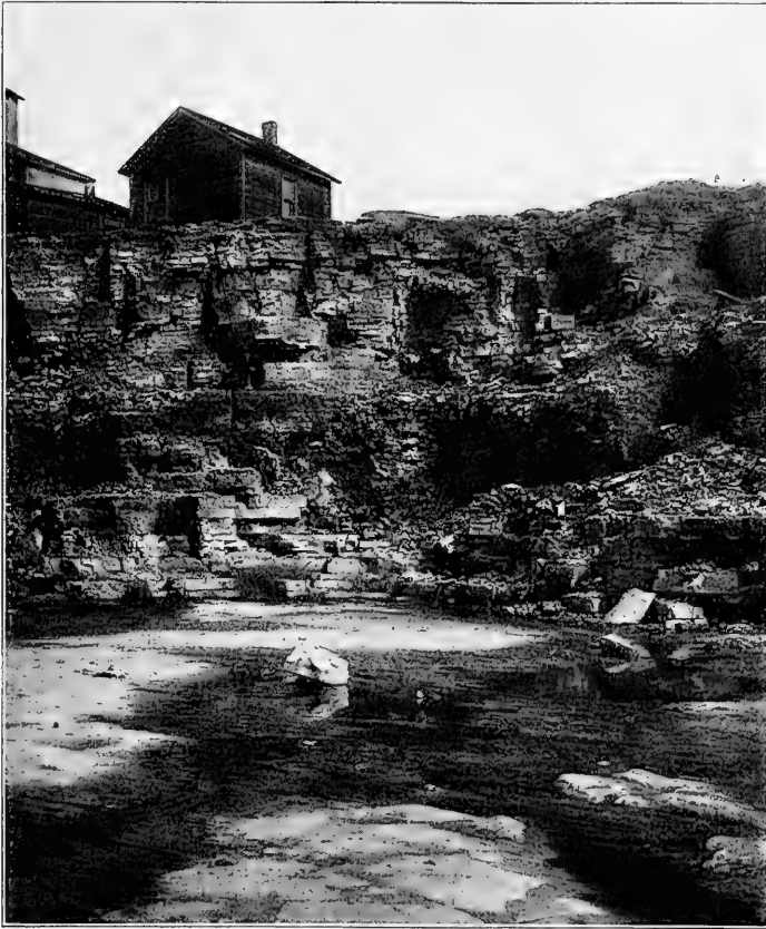
FIG. 1.—Eastern wall of the Jackson Stone Co. quarry, two miles south of Covington, Ohio. The lower part is the Laurel limestone. Mr. Cottingham's foot is on top of the "mottled zone," above which is all of the Springfield dolomite, while the top of the wall is the base of the Cedarville dolomite.
