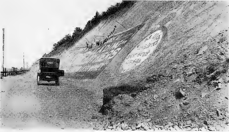
FIG. 5.—Slickenside surface exposed along road cut in north end of Plum Ridge. (Photo by J. P. Buwalda.)
