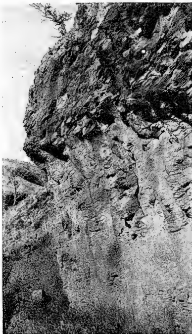
FIG. 14.—Bent columns. (Jackson's Creek, Sydenham, Australia.)
