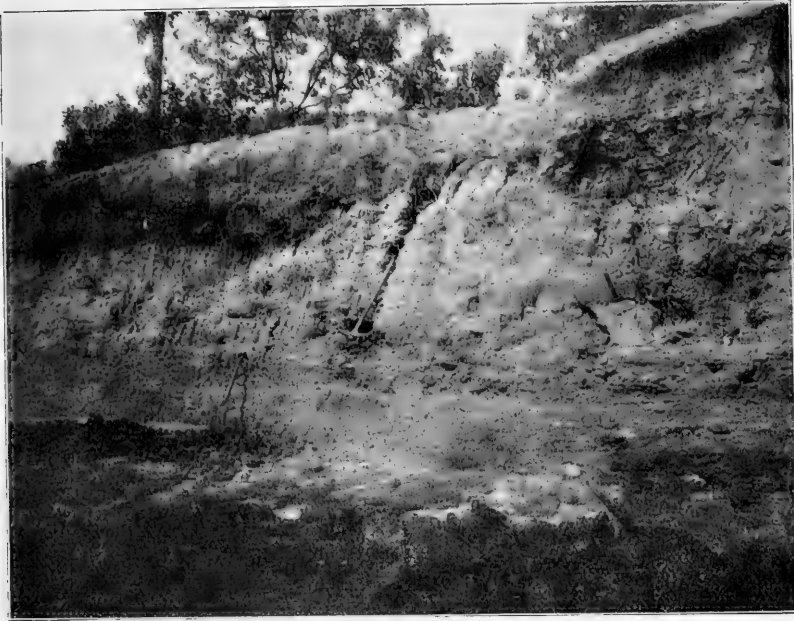
FIG. 2. View in western part of Green quarry north of Platte River at Louisville, showing line of unconformability between Dakota sandstone and Carboniferous limestone. The hammer marks the limestone, No. 3 of section, on which the Dakota sandstone rests, and only three feet to the west, marked by the pick, the limestone is wanting and the Dakota rests on shales of No. 2.
