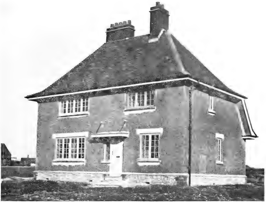
FIG. 9.—Cottage in Chalk Cob. Completed. Front View.
