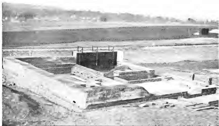
FIG. 1.—Pisé de terre walls on brick base. Shuttering in position on wall. (Author's pattern).
