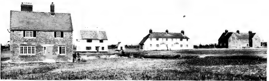
FIG. 8.—Amesbury. General view. Left to right: Cottage in Brick; Cottage of proprietary Concrete Blocks; pair of Cottages in Brick, whitewashed; and pair of Cottages in Brick.
