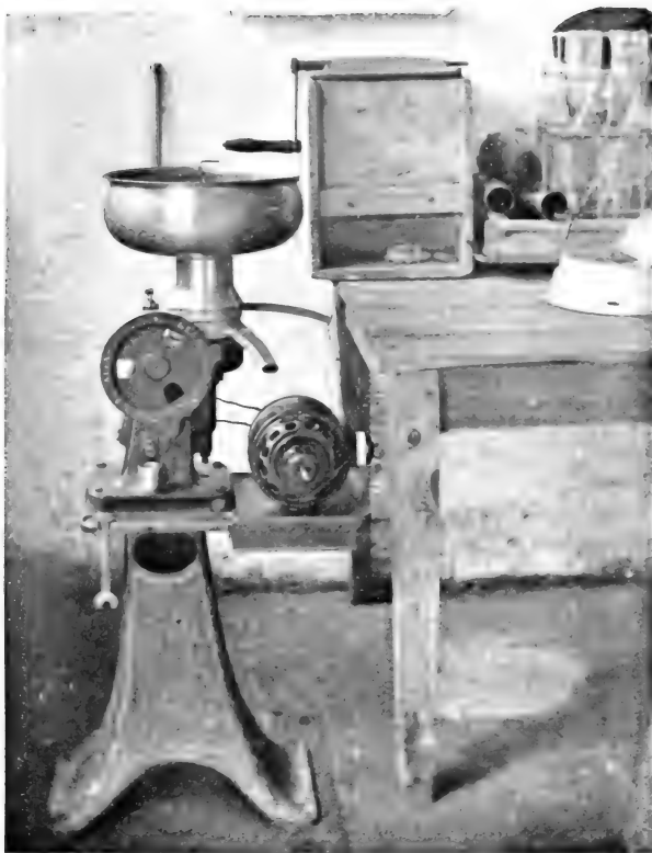
FIG. 1.—An electrically-driven Cream Separator at Greater Felcourt Farm.
