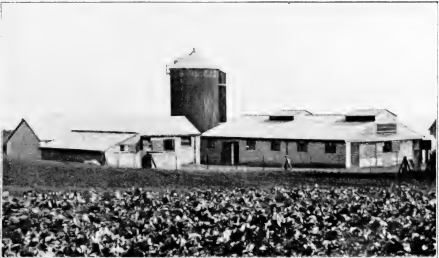
General View from South-West.
