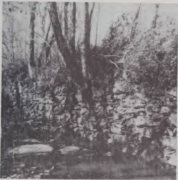
Rock milldam at Iron Works. Probably built in the 1780's. Photo by the author.
