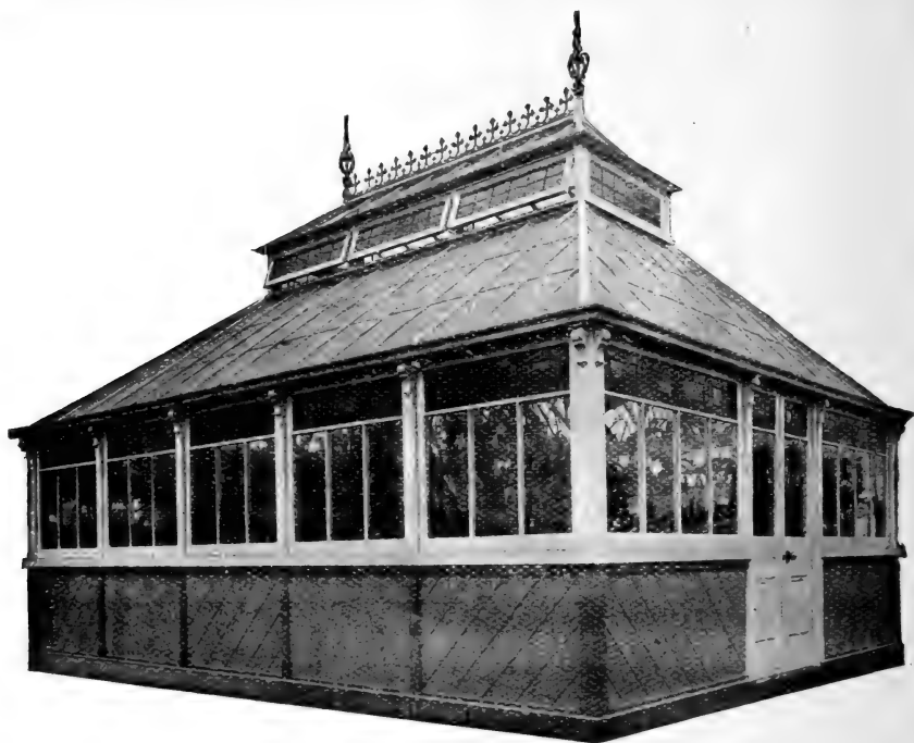
Erected at Bath and West of England Show, Bristol, 1903.
