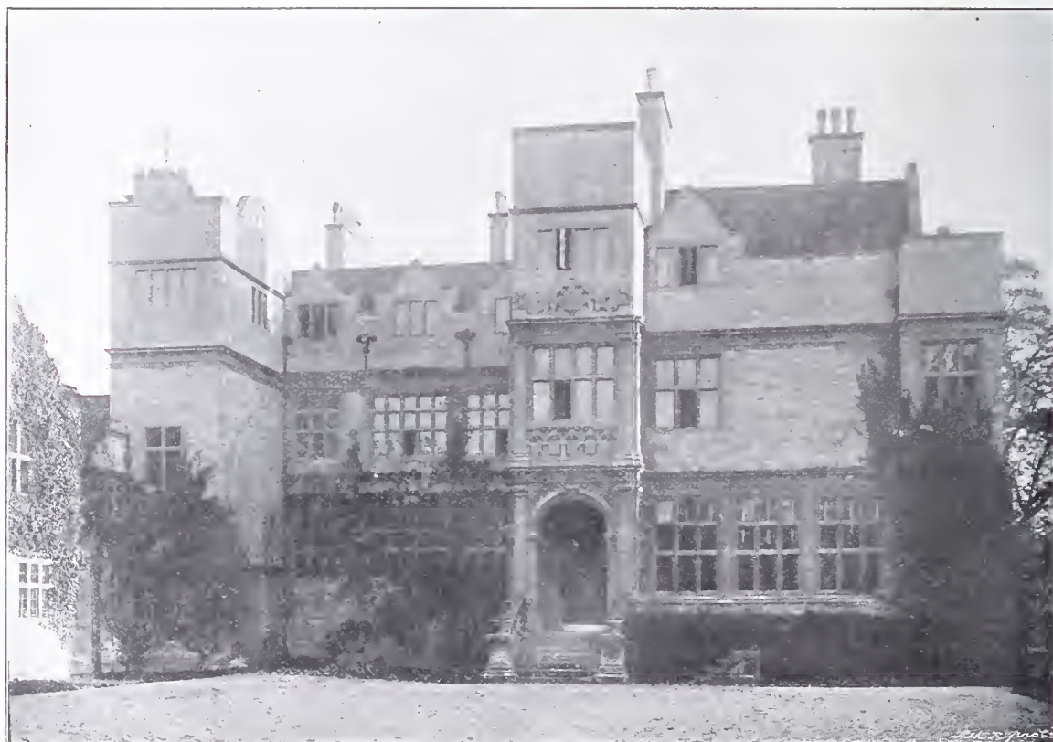
FIG. 4.—LECHLADE MANOR: ENTRANCE FRONT (1872-73).
