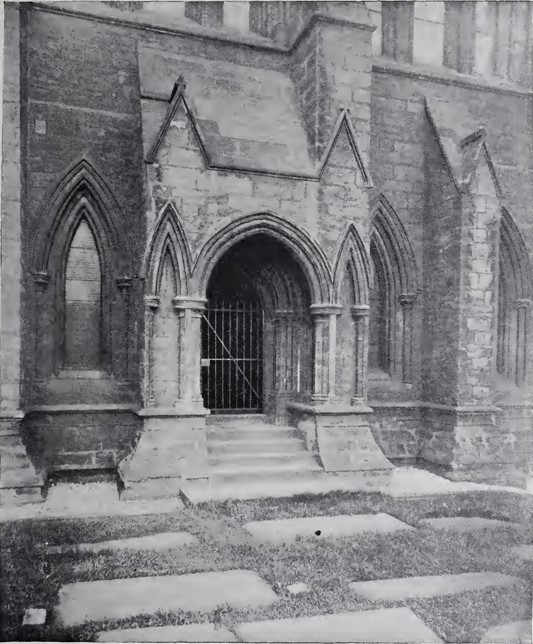
Fig. 2.—SOUTH DOORWAY OF LOWER CHURCH (ROB ROY DOORWAY.)
