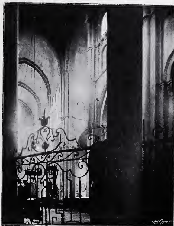
FIG. 7.—PARAY-LE-MONIAL. FROM SOUTH-EAST.
