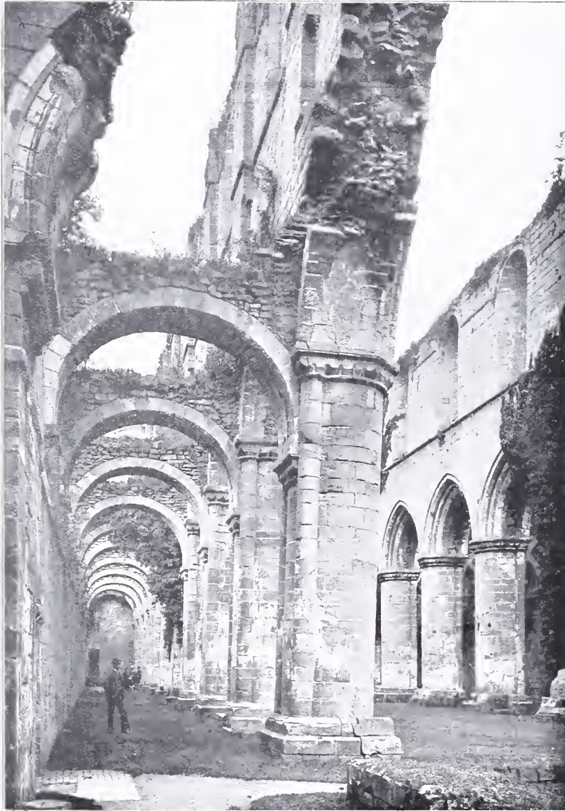
SOUTH AISLE OF NAVE.
