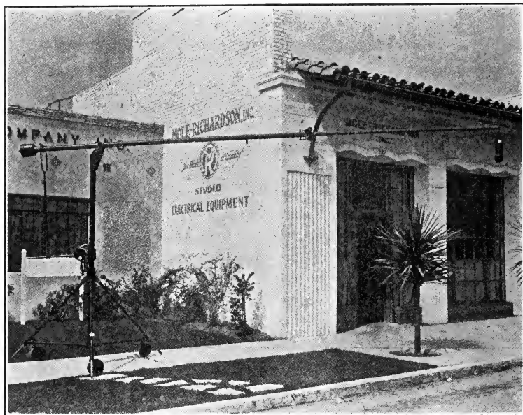
FIG. 1. Microphone boom designed by Metro-Goldwyn-Mayer.
