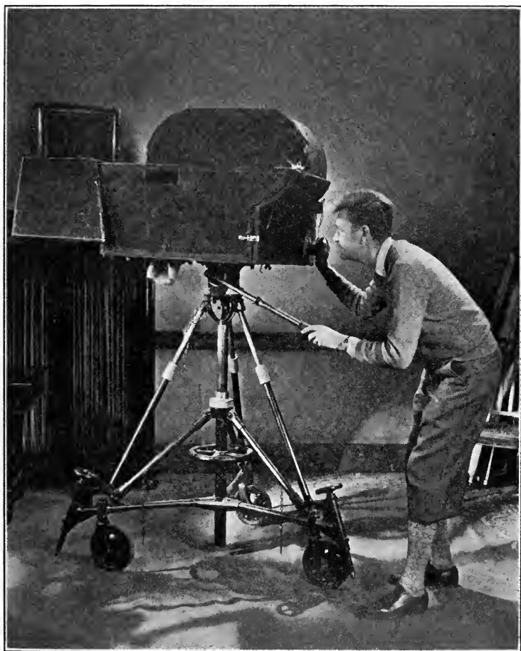
FIG. 6. Rolling tripod modified for lighter blimps.
