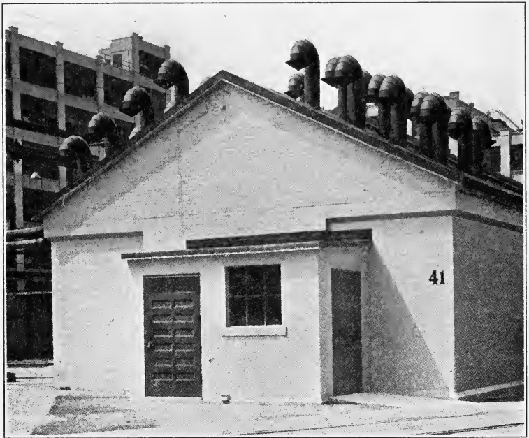
FIG. 11. Exterior view of vault showing ventilators protruding through the roof.
