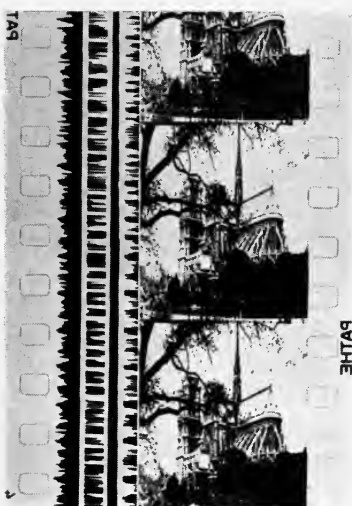
FIG. 3. Combination of the anamorphic image and the three sound tracks.
