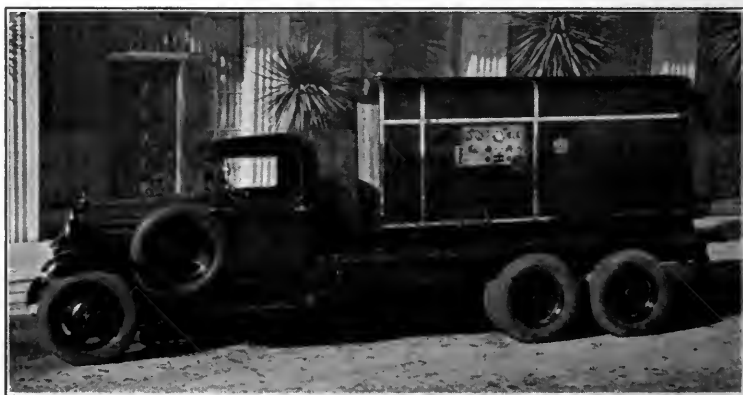
FIG. 3. 160-kw., gas-electric generator set.
