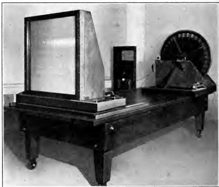
FIG. 6. View of the projection apparatus from the front, showing the projecting lens and the rod screen.
