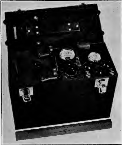
FIG. 2. Amplifier assembly showing cover raised.
