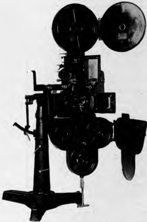
FIG. 22. Double-film preview attachment for projectors ( RCA, Ltd. ).
