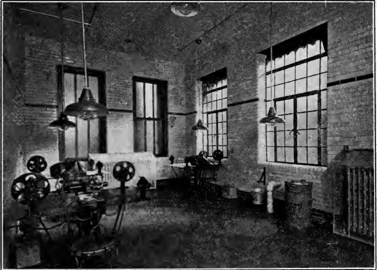
FIG. 2. Inspection room, St. Louis (Mo.) exchange. Note the mesh screen over the radiators, sand pail, vapor-proof lights, sprinklers, metal window frames, metal chairs and tables, side-wall pilot lights, scrap film container. The room has two exits, one into the shipping room and another into an alley.
