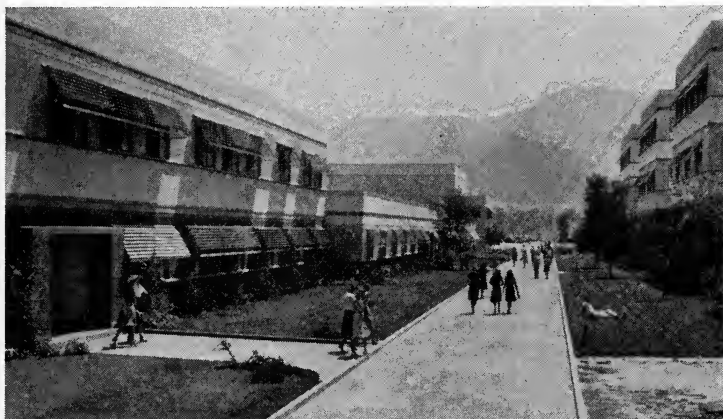
FIG. 2. View down "Minnie Mouse Blvd." showing, on the left, Inking and Painting, Camera, Cutting, Shorts, and Live Action Buildings, and on the right the Animation Building.
