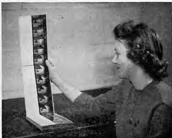
Fig. 3. Cardboards to which description and enlargements from individual motion picture frames are attached and which are joined by tape hinges. The action of locking of the 20-mm aircraft cannon may be studied picture by picture.
