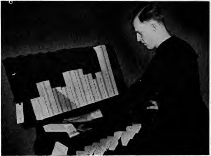
FIG. 3. Sequencing punch cards on the sorting machine.
