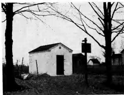
Fig. 3. Coaxial cable auxiliary repeater station.
