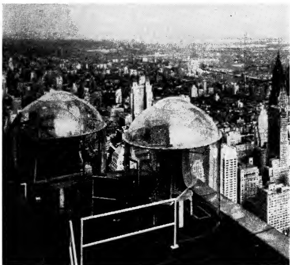
Fig. 6. Local channel microwave equipment on Empire State Building.
