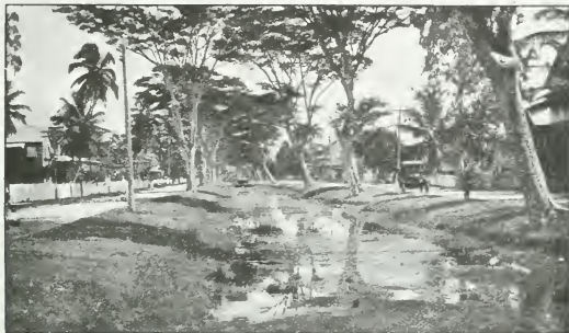
FIG. 1. — Street drain before filling.
