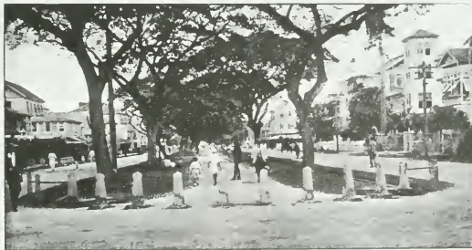
FIG. 2. — Street drain after filling.
