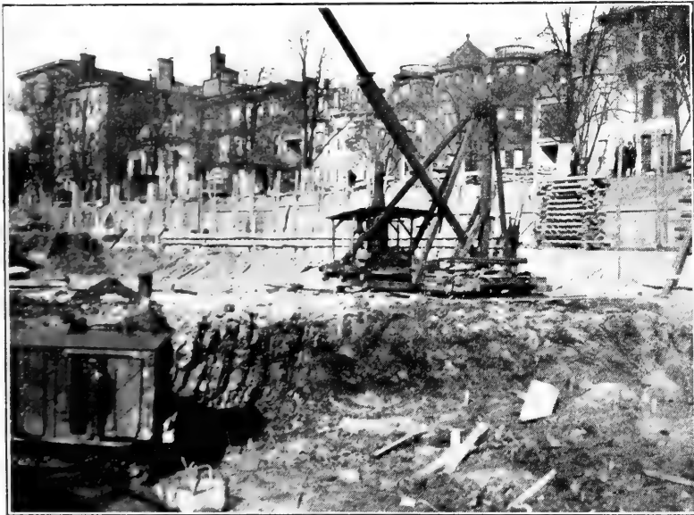
Fig. 6. View showing the edge of the swamp deposit into which the steam shovel is cutting. The form of a mud covered cypress stump upright and in place in the muck is indistinctly shown just to the right of the overturned bucket.
