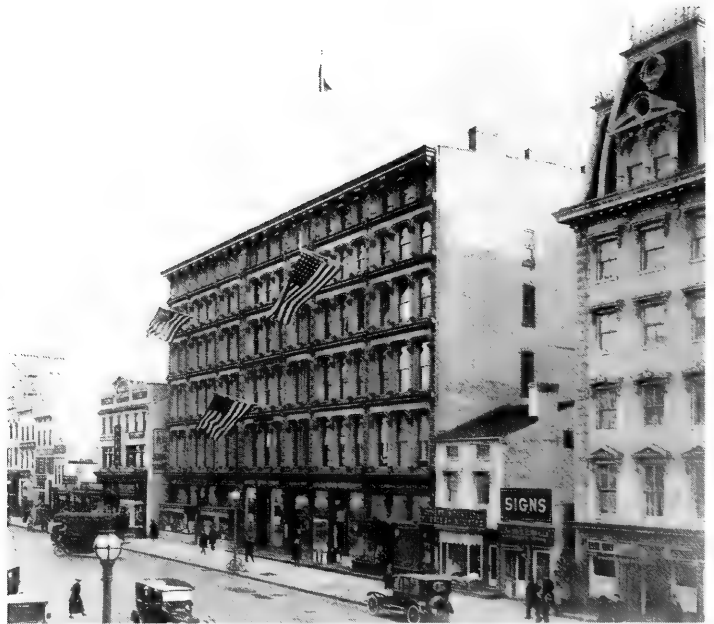
Figure 22. The Hooe Iron Building at 1324-1334 F. Street N. W. in Washington, D.C., where the "National Center" of the U.S. Geological Survey was housed from 1884 to 1917, next to the "new" Ebbitt Hotel.
