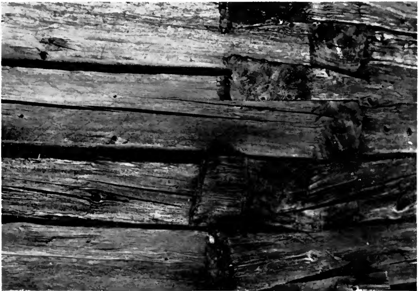
Plate 9. Detail showing manner in which church logs were fitted.
