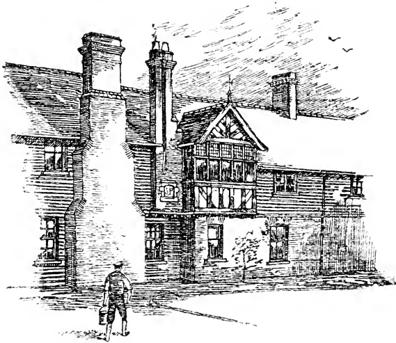
PORTION OF PARK HOUSE, SOUTH VIEW
