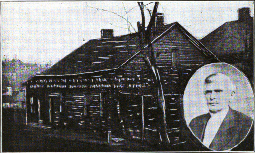
FIRST M. E. CHURCH BUILDING IN CADIZ, O., COR. BUFFALO AND SPRING STS., BUILT ABOUT 1816. BISHOP MATTHEW SIMPSON PREACHED HIS FIRST SERMON HERE.
