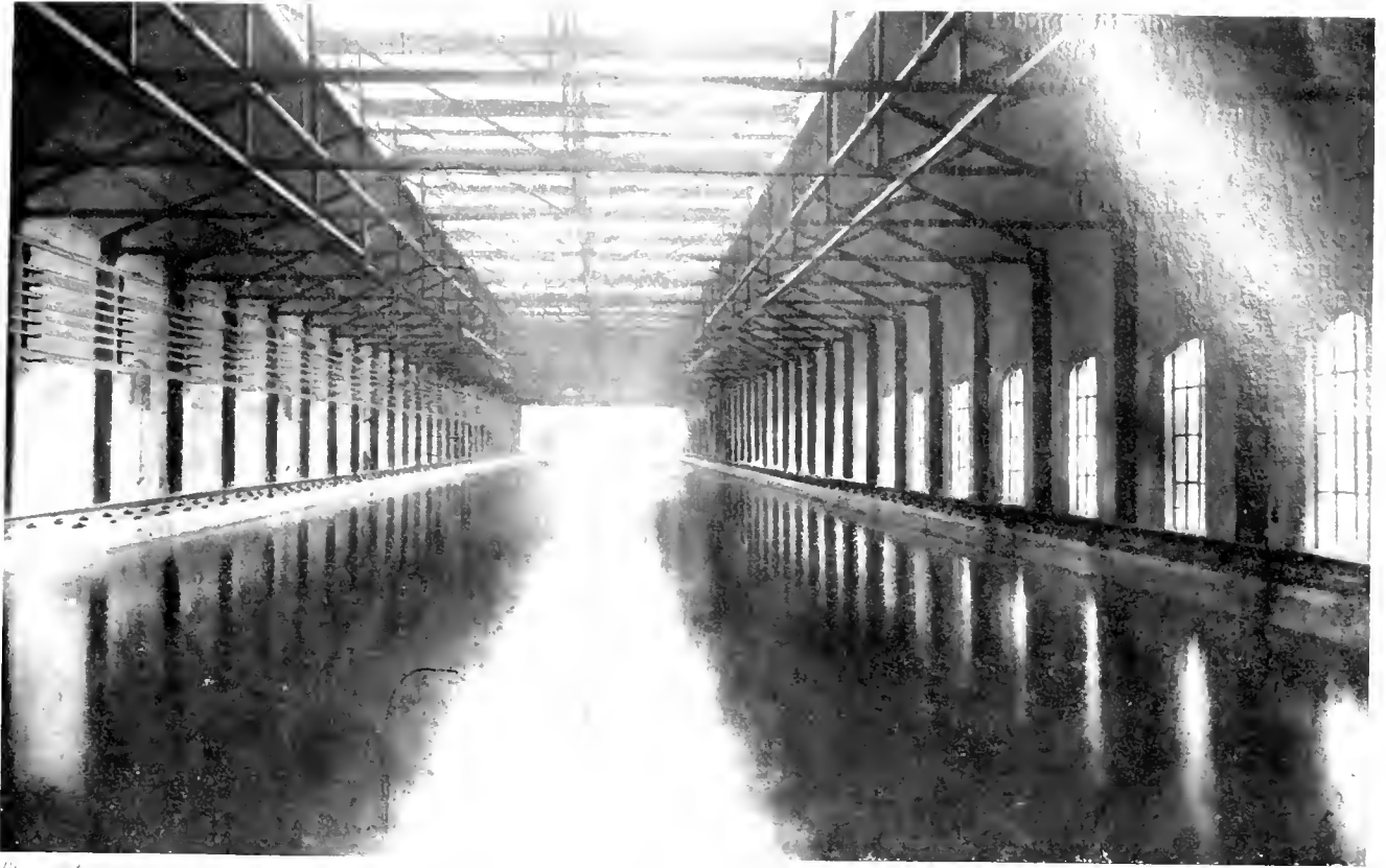
FIGURE 4. General View of the Experimental Tank.
