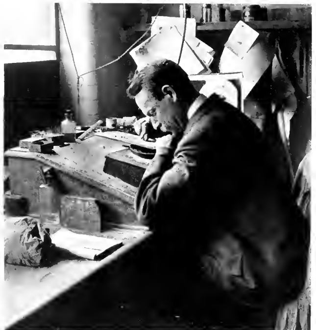
FIGURE 10. Engraving the Plate. "Taking out blemishes."
