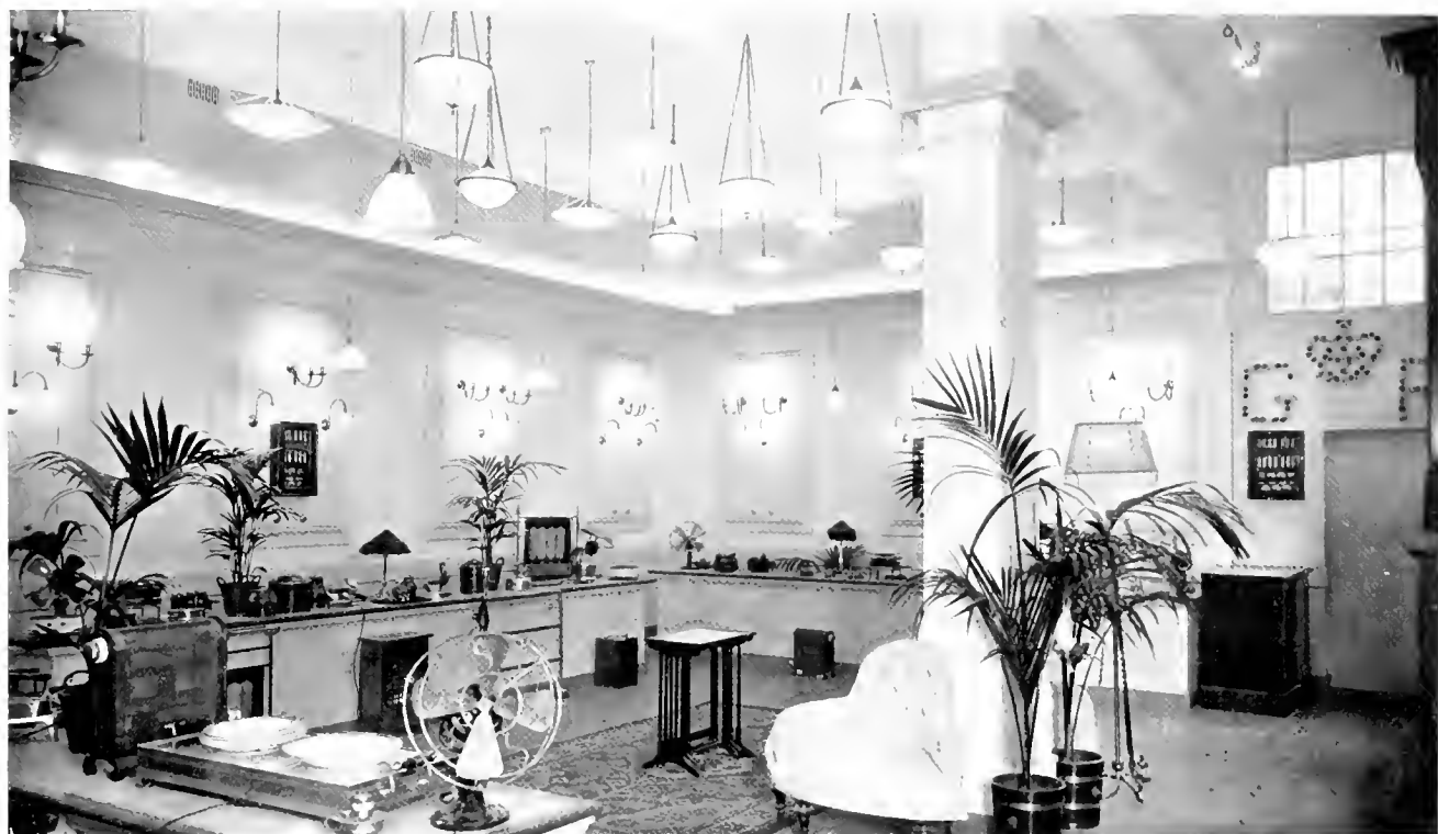
Demonstration Room at the Westminster Electric Supply Corporation.
