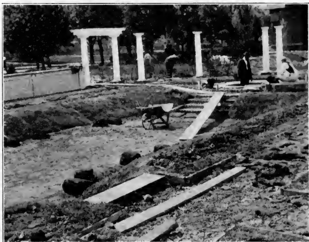
Fig 3—Garden in construction, showing grading to conform with steps and walks
