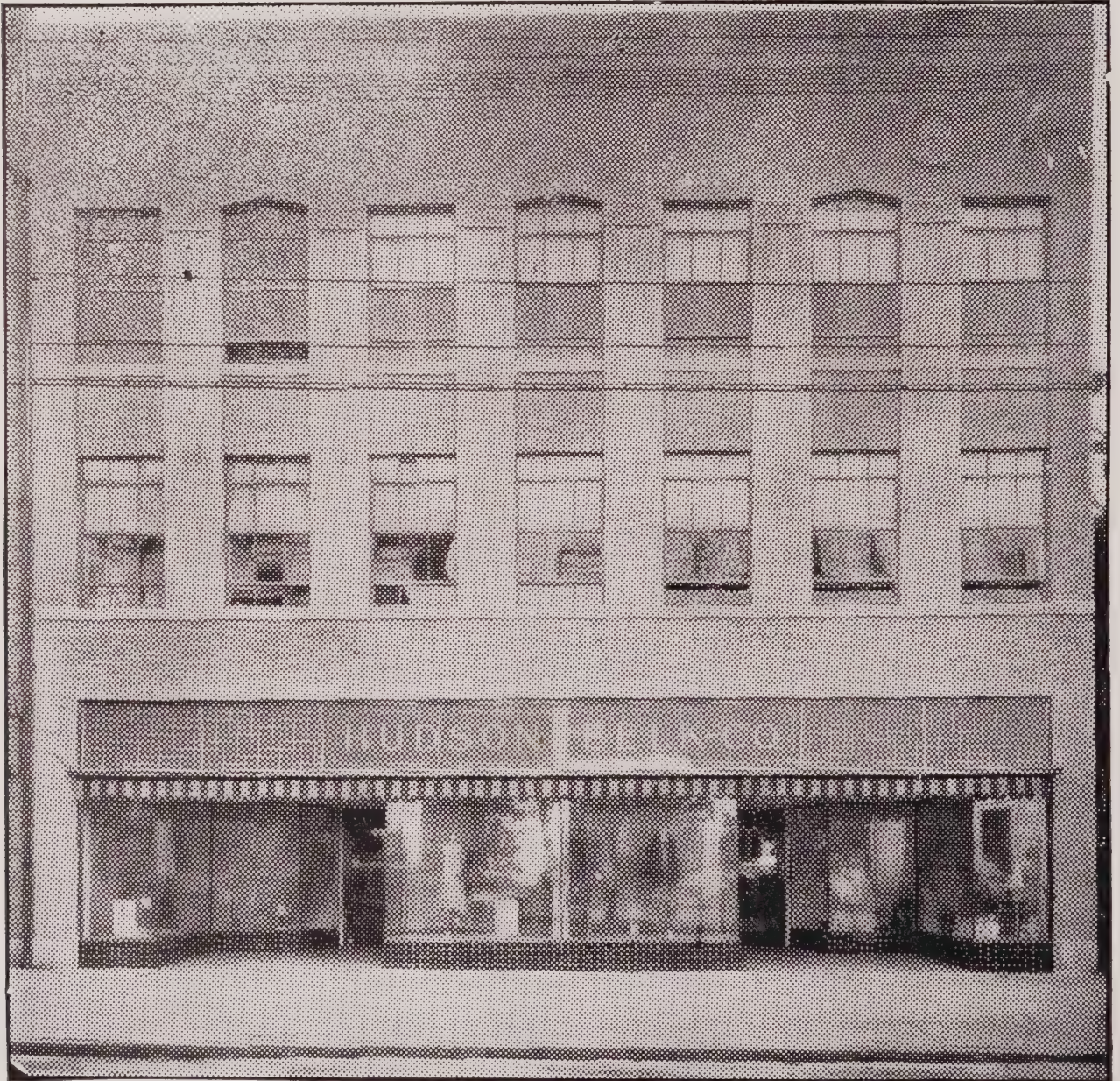
Fayetteville Street entrance of the new home of Hudson-Belk Department Store, now one of the largest most modernly equipped of such buildings in Eastern Carolina.
