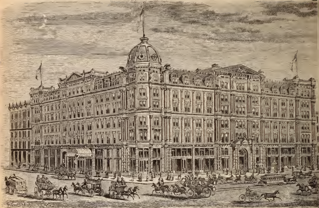
FIG. 183. Palmer House, Chicago, Illinois.
