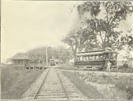
BACK RIVER STATION MONTREAL PARK AND ISLAND RAILWAY.
