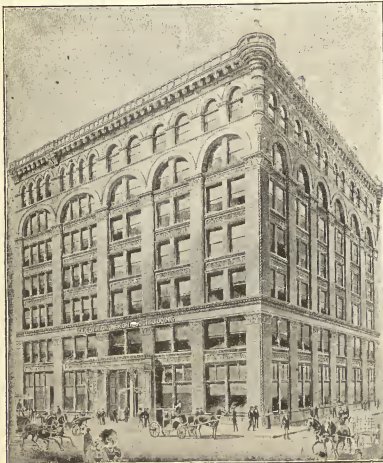
Electrical Exchange, Liberty and Washington Sts., New York.
