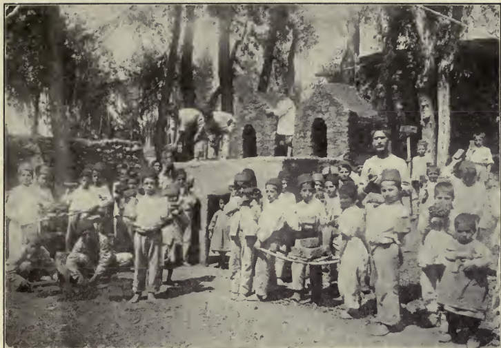
ORPHANS LEARNING TO BUILD HOUSES, VAN
