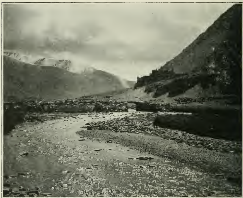
Bridge over the Nyang chu above Kang-ma.
