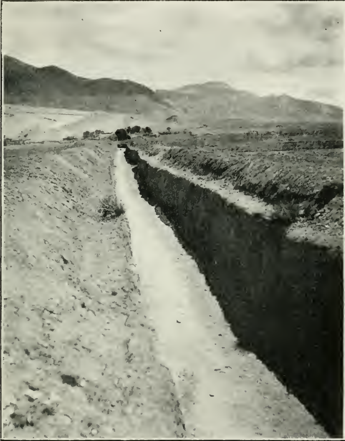
The covered way constructed by Captain Sheppard between Chang-lo and Pala
