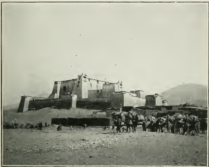
Phari Jong. The hole in the wall afterwards increased in size.
