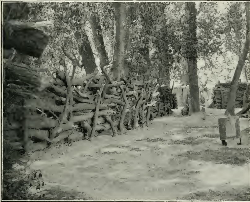
Traverses of timber built for the protection of Chang-lo.
