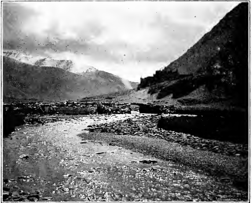
Bridge over the Nyang chu above Kang-ma.
