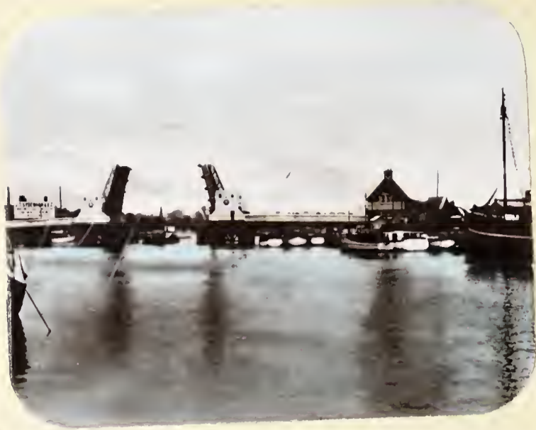
Hamworthy Bridge (Open), Poole.
