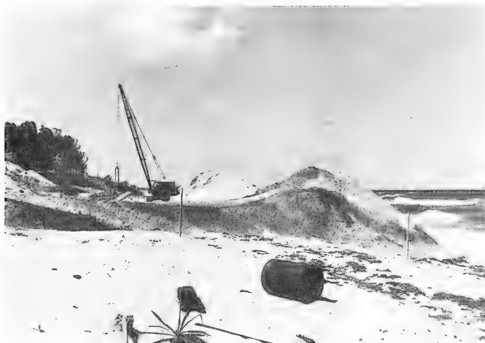
Figure 7. Dune leveling at Boca Raton site, 7 May 1969; midtide, falling ( H = 3.4 ft, T = 3.6 s, \alpha_b = 2^\circ ).
