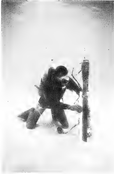
Figure 17. Diver making subaqueous sand level measurement at the Boca Raton site.
