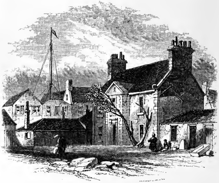
WATT'S HOUSE, DELFTFIELD LANE.
