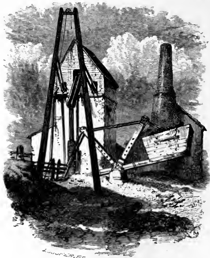
CARDOZOS PUMPING-ENGINE, UNITED MINES.
