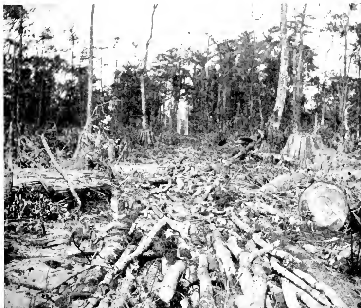
FIG. 103. — The Pole Foundation for a Dunnage Road in a Cypress Swamp, Louisiana.
