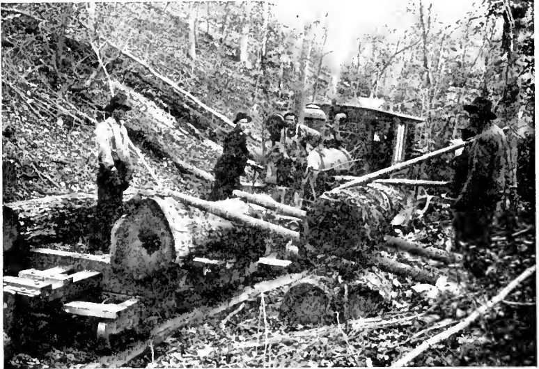
FIG. 98. — A Stringer Road in the Appalachian Mountain Region.
