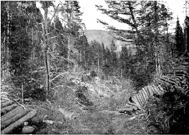
FIG. 25. — Skidways along a Two-sled Road. Montana.
