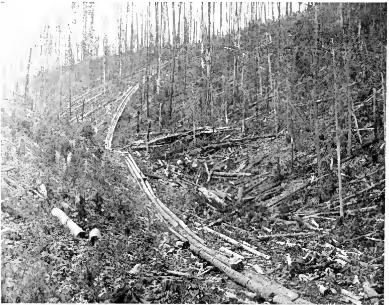
FIG. 84. — A Two-pole Running Log Slide. Idaho.
