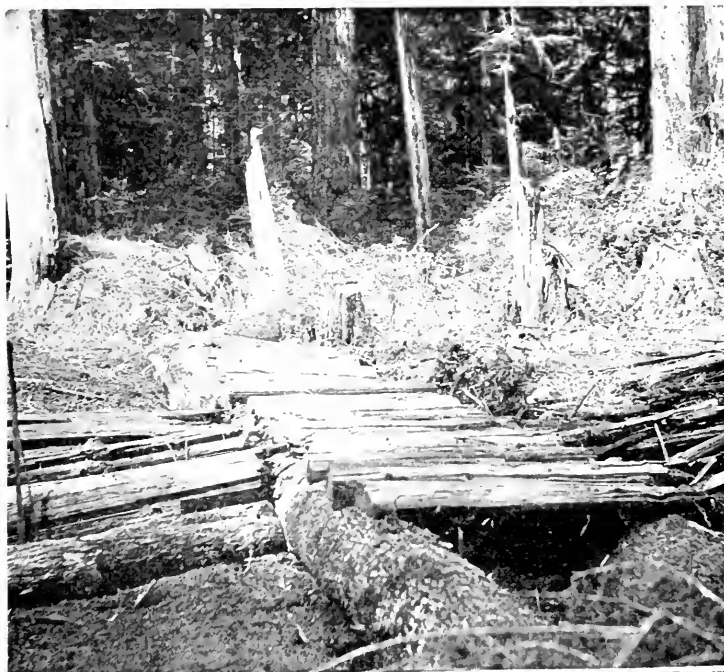
FIG. 106. — A Culvert on a Logging Railroad Spur ready for the Earth Cover. Note the use of non-merchantable material for filling depressions on both sides of the culvert. Washington.
