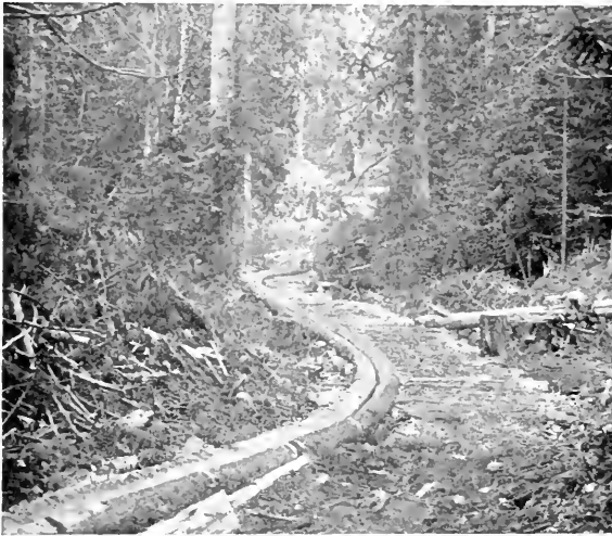
FIG. 85. — The Lower End of a Trailing Log Slide. Note the corduroy bottom over which the tow team travels. Idaho.
