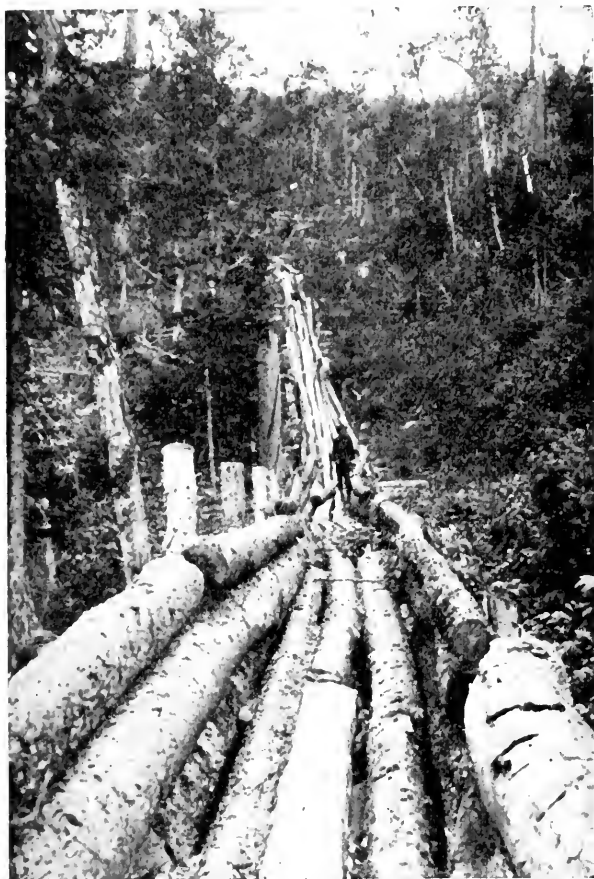
FIG. 92. — A Timber Chute for bringing Logs down Steep Slopes. New Hampshire.
