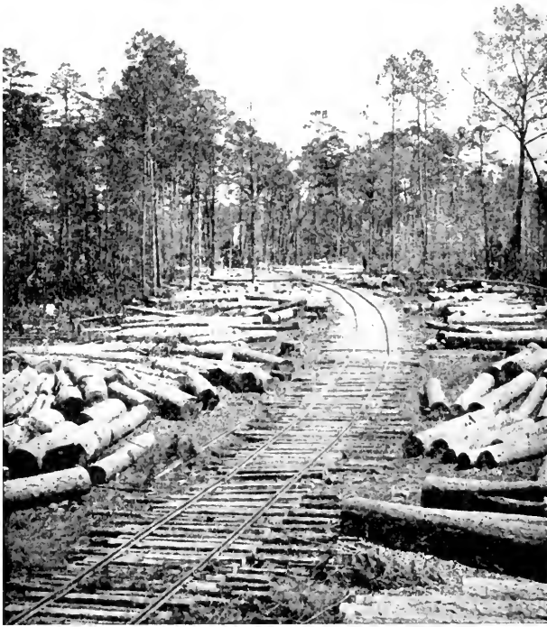
FIG. 105. — A Spur Logging Railroad Corduroyed with Poles in order to provide an Adequate Bearing Surface on a Soft Bottom. Arkansas.
