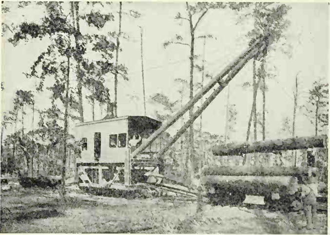
FIG. 124. — The Decker Log Loader.
