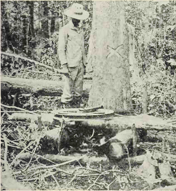
FIG. 75. — A Sheave Block attached to a Tail Tree on a Pullboat Operation. Note the method of supporting the block; also the cross on the tree which denotes its selection as a tail tree.
