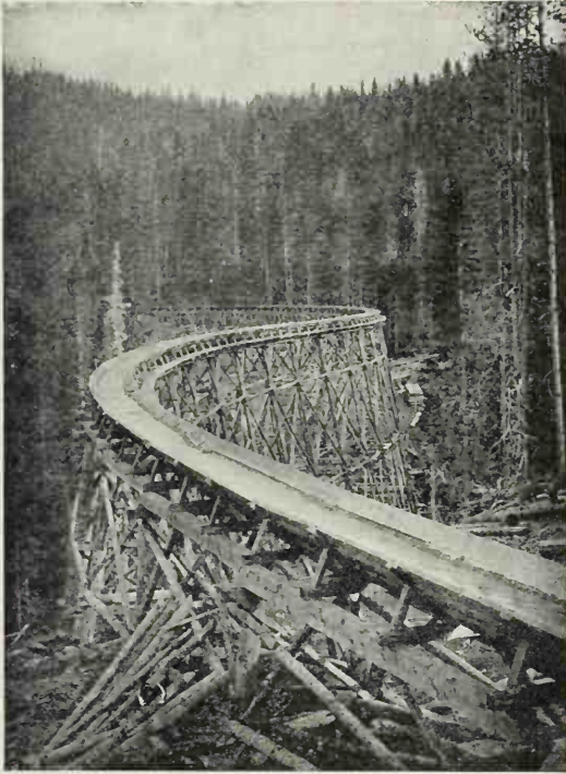
FIG. 159. — A V-flume for transporting Mining Stulls. Montana.
