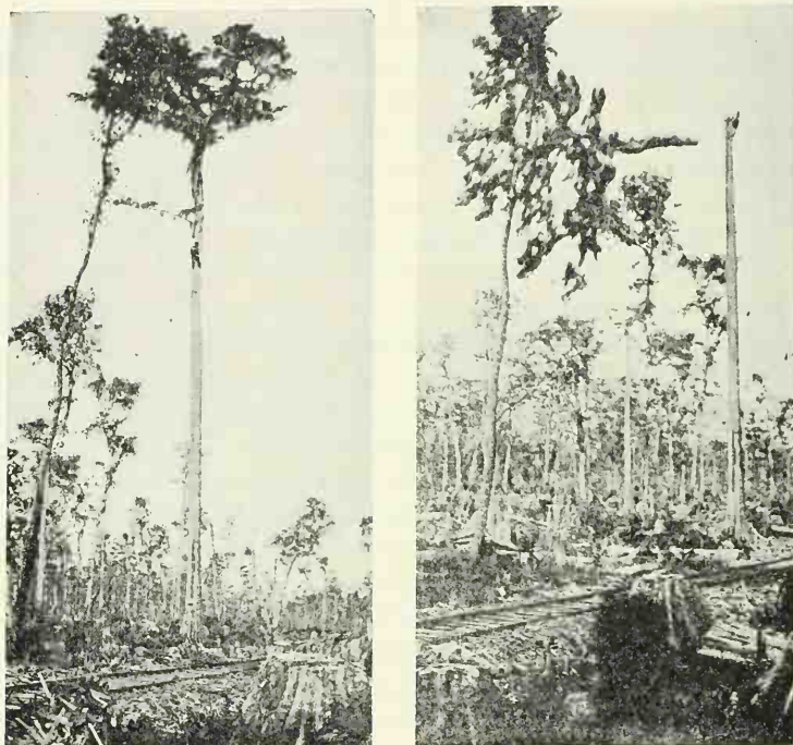
FIG. 65. — Cutting the Top from a Head Spar on which is placed the Main Cable Rigging for a Cableway Skidder. Cypress Forest, Louisiana.
