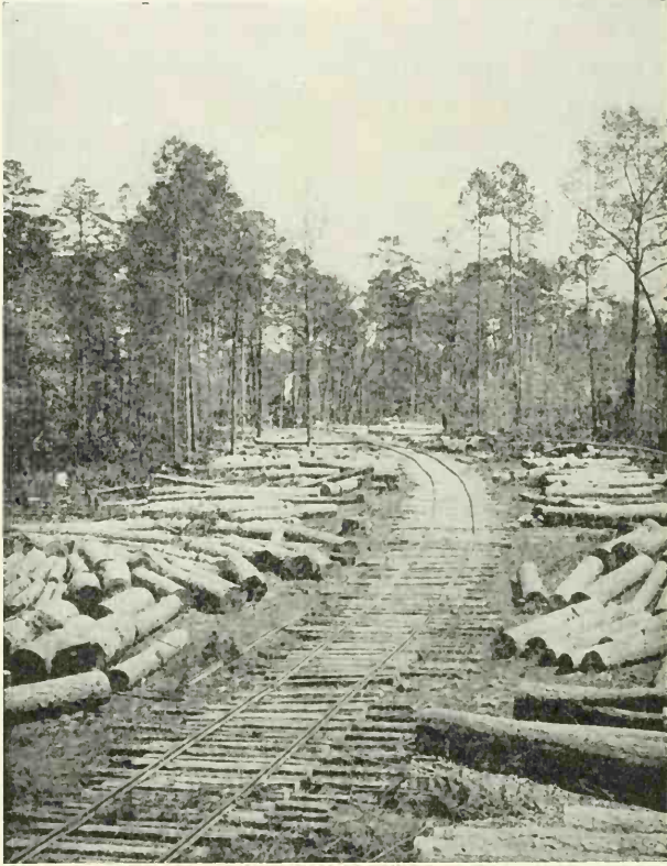
FIG. 105. — A Spur Logging Railroad Corduroyed with Poles in order to provide an Adequate Bearing Surface on a Soft Bottom. Arkansas.
