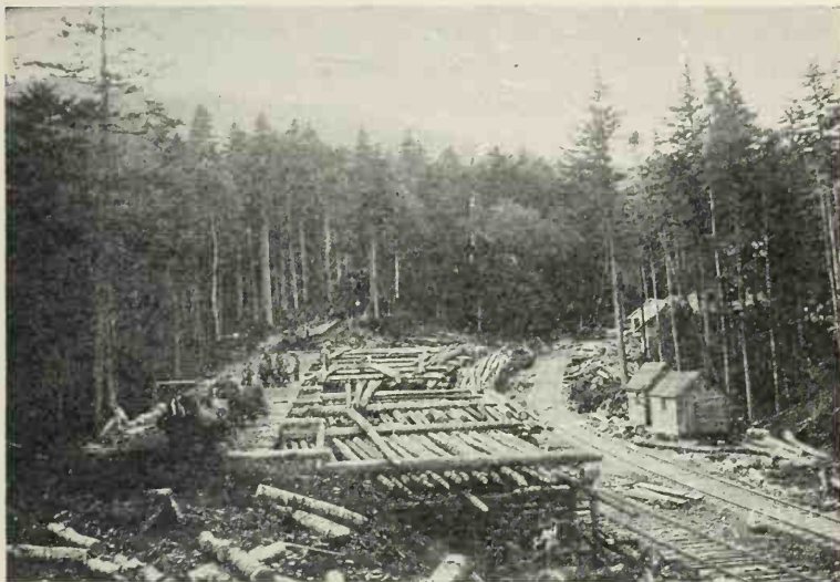
FIG. 27. — A Skidway or Loading Dock along a Logging Railroad in West Virginia. The logs in the structure are later loaded and hauled away.
