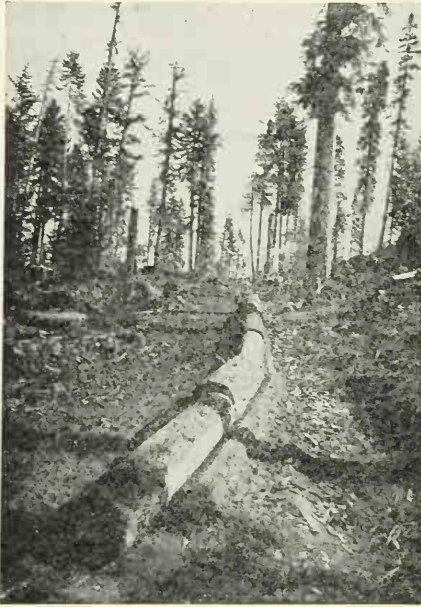
FIG. 91. — A Fore-and-aft or Pole Road used with a Road Engine. Pacific Coast.
