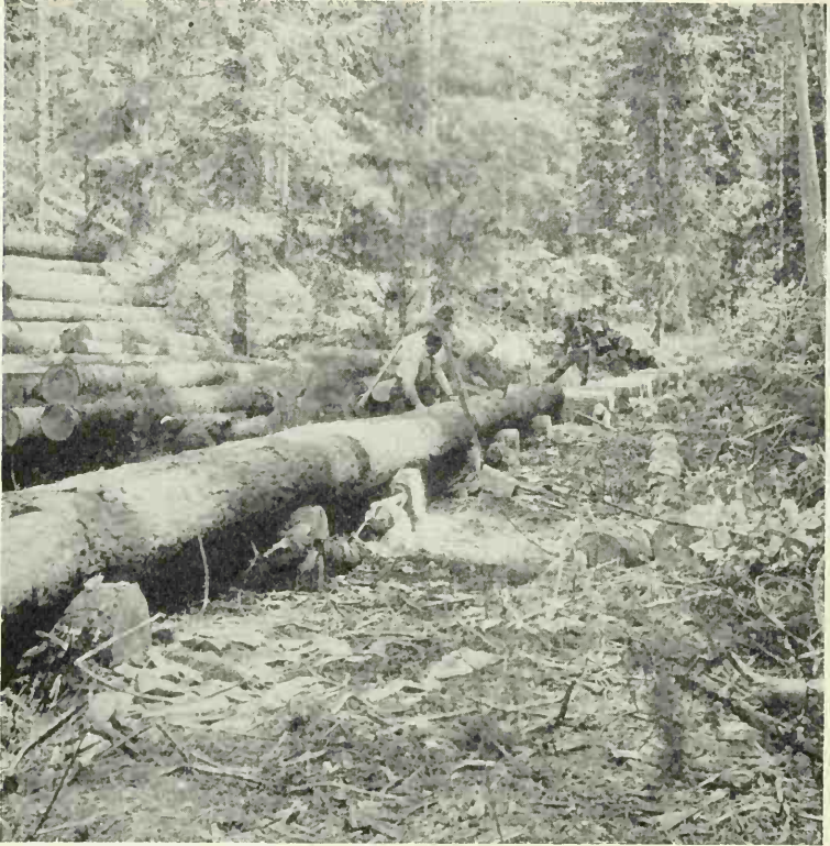
FIG. 86. — A Trailing Two-pole Log Slide in process of construction. Idaho.
