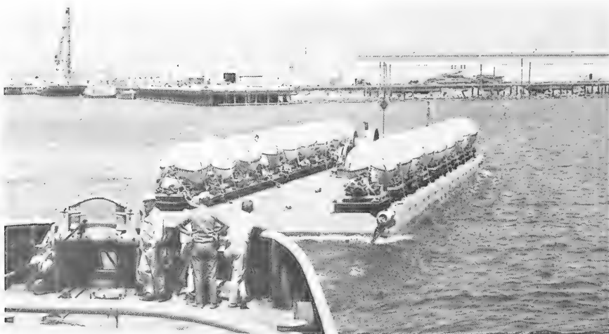
Figure 7. Spheres rigged on barge in preparation for free-fall launch.
