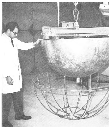
Figure 2. Arrangement of steel bar reinforcement for Spheres 17 and 18.
