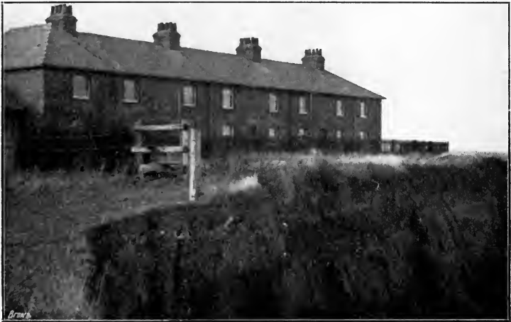
THE COTTAGES AT SAND-LE-MARR, NOW AT THE CLIFF EDGE.
