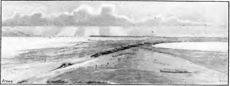
NEAR KILNSEA BEACON, LOOKING SOUTH: SHOWING THE FLOODED AREA, 1906.
