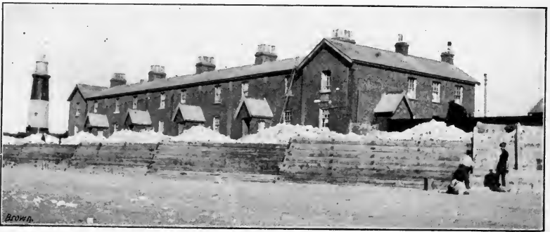
THE HOUSES AT SPURN, SHOWING METHOD OF PROTECTING AGAINST EROSION.
