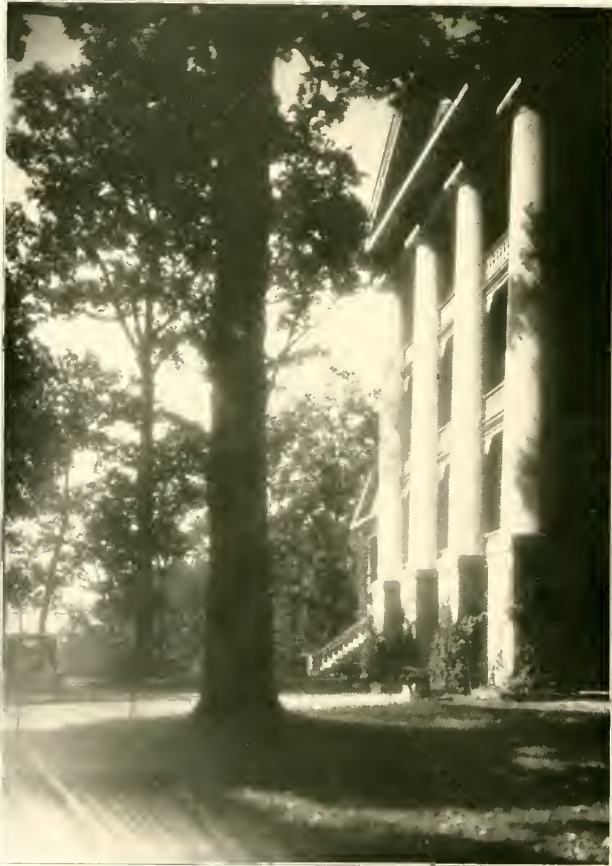
MAIN BUILDING (SIDE VIEW)
