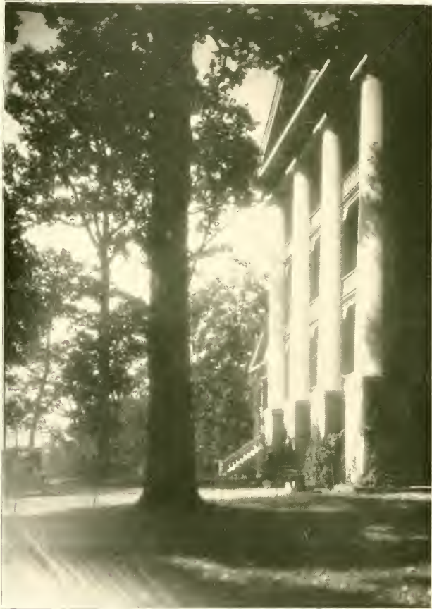
MAIN BUILDING (SIDE VIEW)
