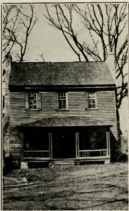
ORIGINAL BUILDING Erected in 1802
