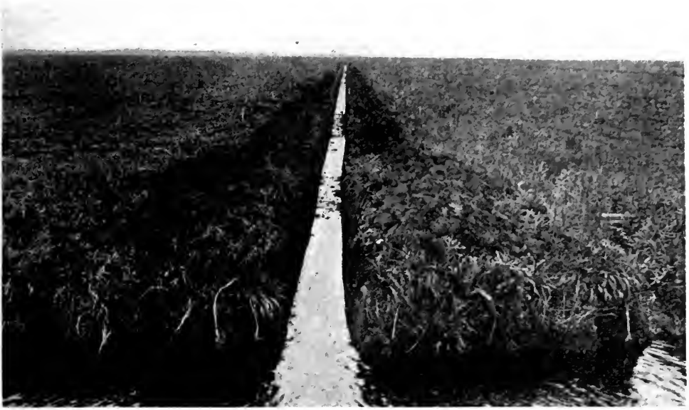
Drainage Canal Entering into Main Canal
