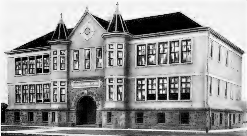
Luther Burbank School, Santa Rosa, Cal.
