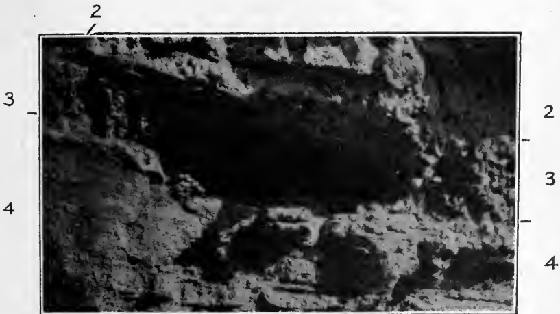
Fig. 5.—View of hole eroded into stratum 3 at nitrate exposure on south side of point. Also shows calcite-lined cavities in stratum 2.
