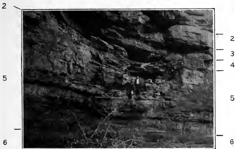
FIG. 3.—View of nitrate-bearing exposure on north side of point, showing weathering into strata Nos. 3 and 5 of the section.
